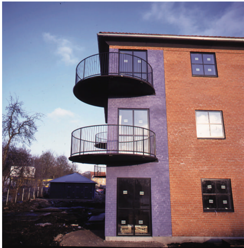
Figure 4 Cantilevered balcony slabs produced in CRC.
