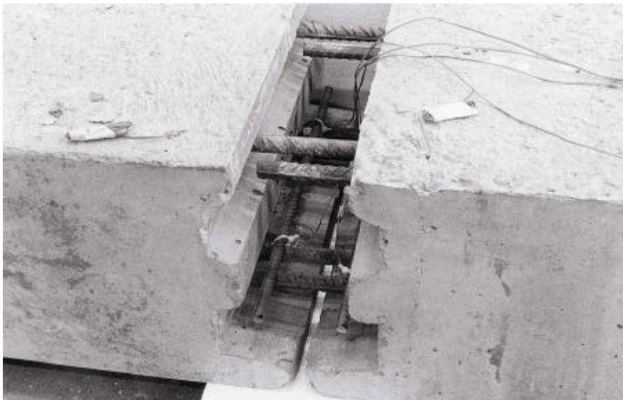
Figure 7 Detail of the joint prior to casting.
